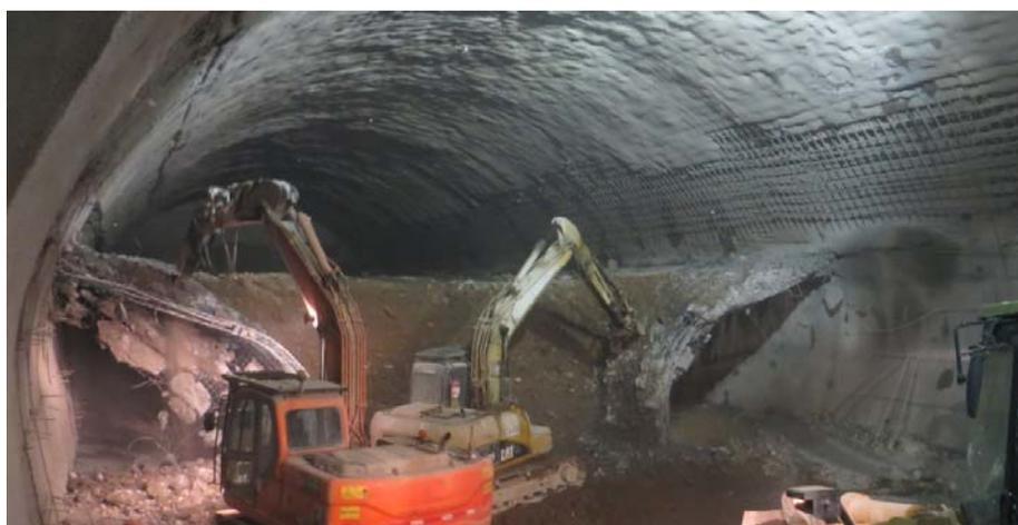
**Photo 3. Bench excavation and demolition of the temporary support of the side-wall galleries.**
