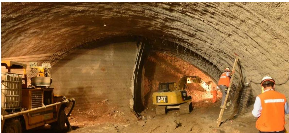
**Photo 1. Vault excavation at Los Leones East Station Tunnel.**
