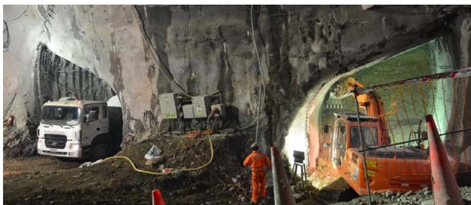
**Photo 2. Side-Wall Foundation Galleries construction at the West part of the Station Tunnel.**
